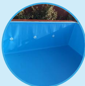
PVC liner cut to the pool
